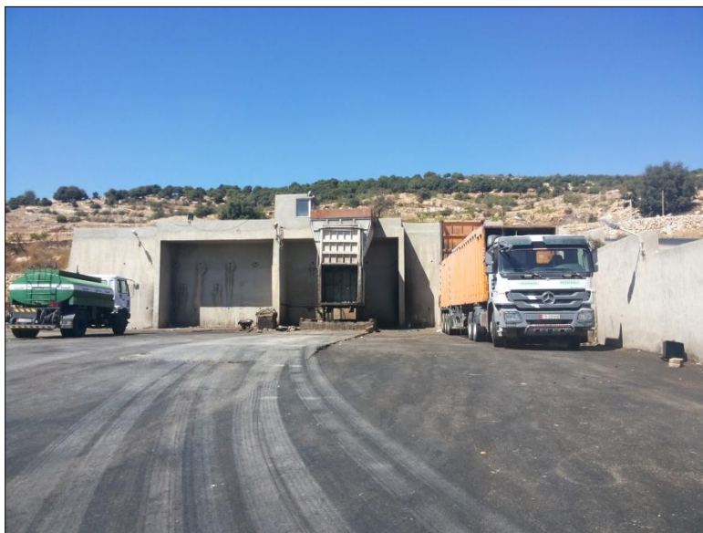
Figure 8: A waste transfer station in good condition
