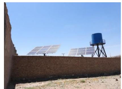
UNHCR's community-based protection programme constructs wells powered by solar pumps to provide safe drinking water to returnee and host communities. © UNHCR/D.Corcoran
