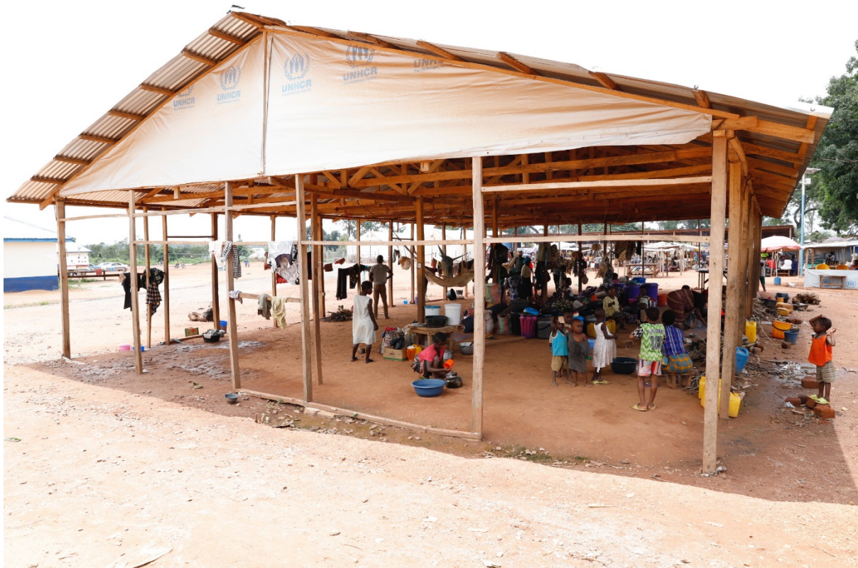
Some 14 refugee families (82 individuals) live under this hangar provided by UNHCR at the Adagom refugee settlement, Cross River State. When it rains at night they have to stand up as the rains flood the floor. © UNHCR/Tony Aseh
