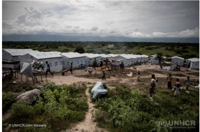
Kasenyi IDP site, Ituri Province, where UNHCR built collective hangars and emergency family shelters to decongest schools and churches. © UNHCR/John Wessels
