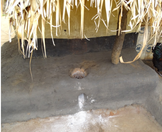
Type of mud-stove constructed in the veranda (host household - Yumbe)
