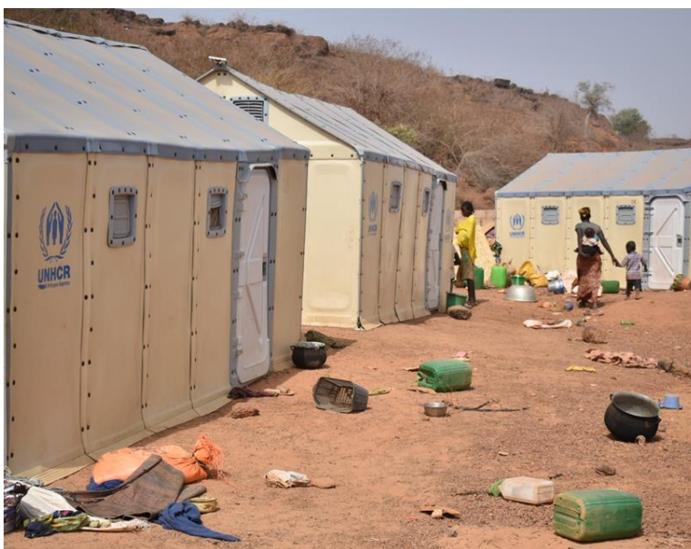
RHUs constructed in Kaya to host IDPs newly arrived from Pensa, following recent attacks that killed 9 civilians. ©UNHCR/M.Bougma
