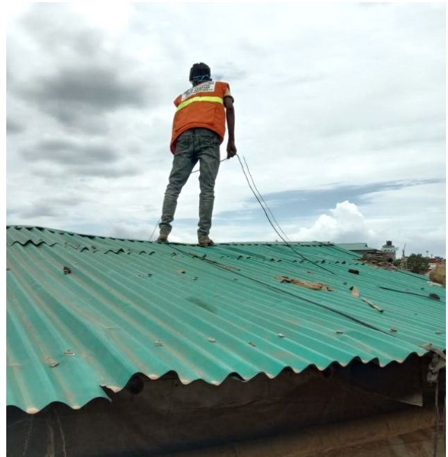
Refugee volunteers using ropes to tie-down rooftops ahead of expected strong winds during the monsoon. Photo: © UNHCR
