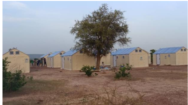
RHUs built in the village of Konkoundi, Centre-North region, benefiting 51 IDPs who occupied the village school. ©UNHCR
