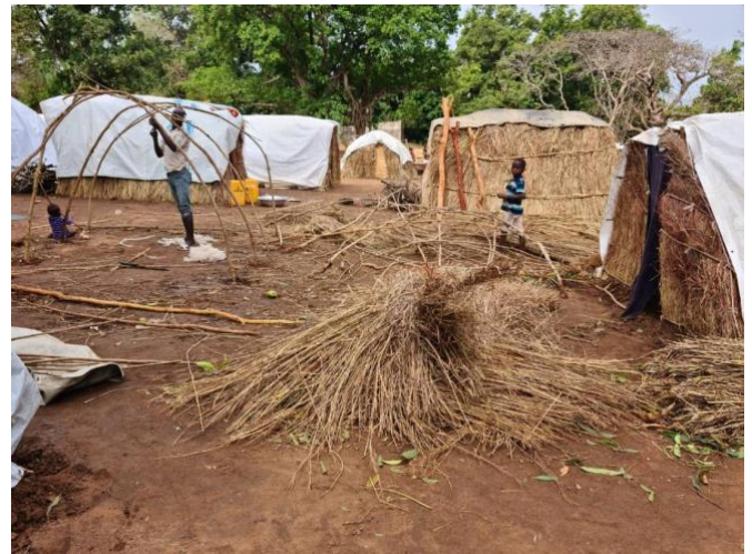
UNHCR assistance to internally displaced persons at a site in Batangafo, Rebuilding lives from branches and a plastic sheet @UNHCR CAR 2021
