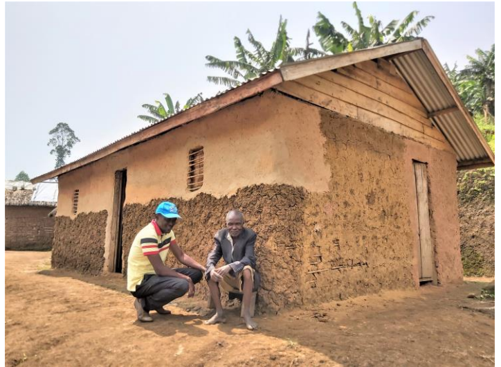
A displaced person and a UNHCR staff member sit in front of a new shelter constructed in North Kivu Province. © UNHCR/Diallo
