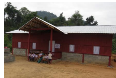
Completed primary school. Photo: UNHCR
