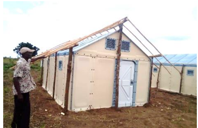
Reinforcing RHUs with wooden posts to increase weather resistance in Bouemba, Republic of the Congo. © UNHCR/Harlette Mafouenta
