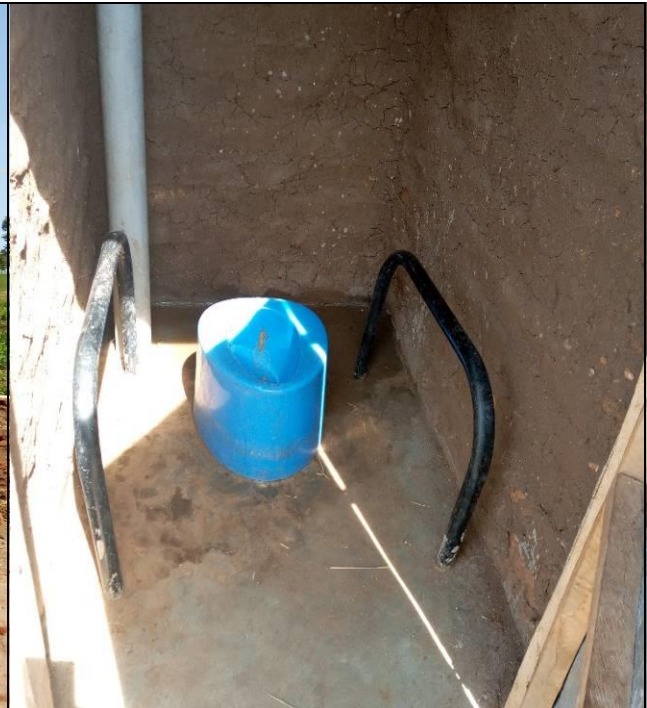
A low cost disability inclusive sanitation facility constructed for PWD household with support from WV
