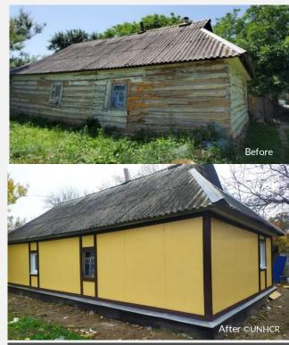
The repair and insulation work for a house damaged by conflict is finished in Kyivska oblast through UNHCR's shelter programme. Before the repairs, the wooden house was vulnerable to the cold and expensive to heat. With the new layer of wall insulation, the house is able to warm the family.
