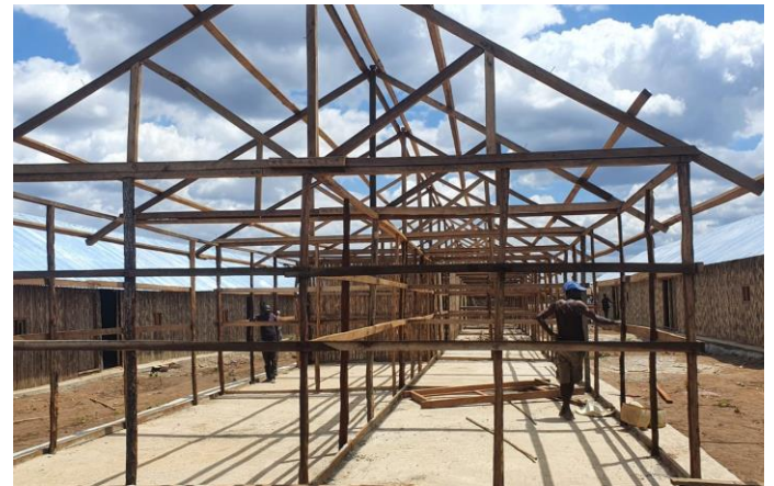
Transit Centre (TC) construction in Lianda IDP site, Mueda ©UNHCR/Gure Abdi
