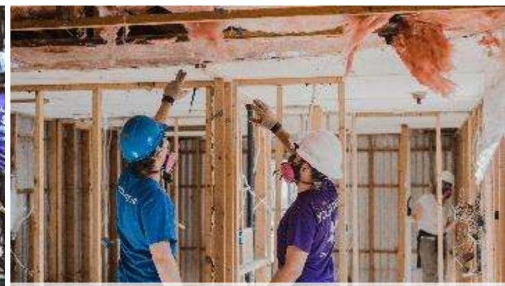
Mucking and Gutting
