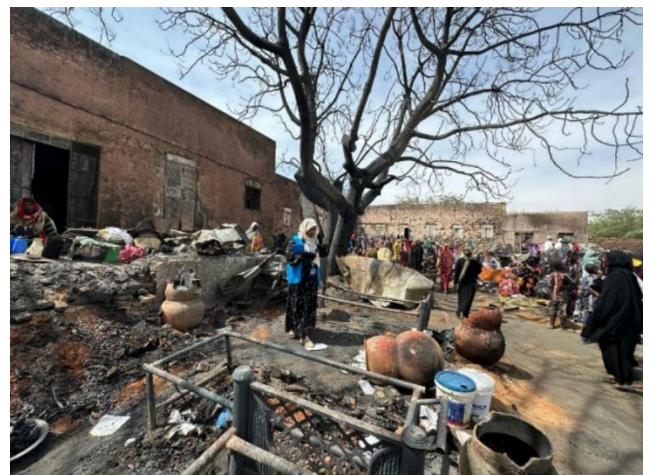
Assessment was conducted after the fire that had broken in West Darfur.
